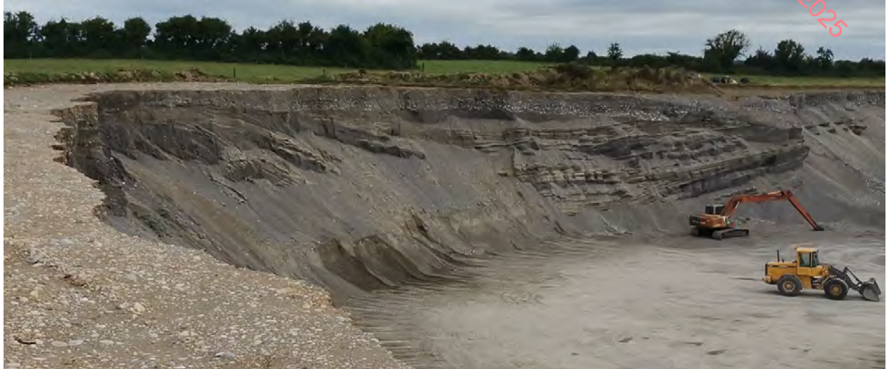
Fig 2.2: View of western working face.
